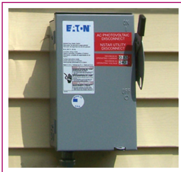
EXHIBIT 690.10 PV system disconnect.
