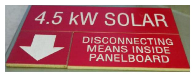
Labels Needed on Solar Installations: System rating/type
